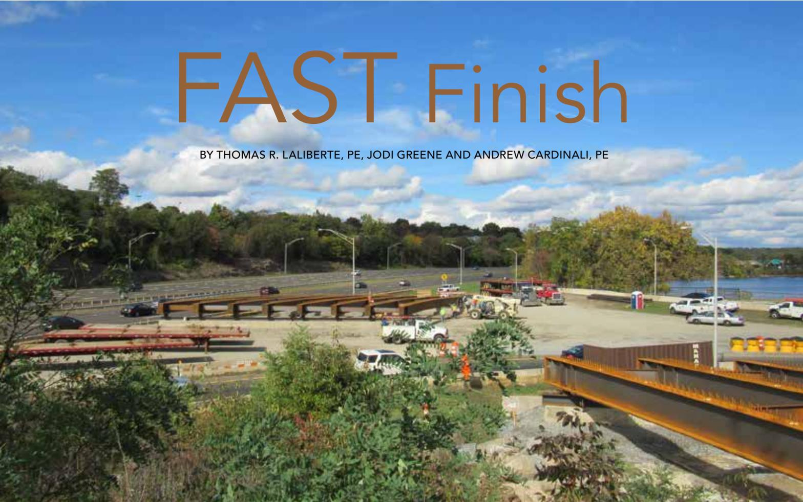
▲ At the lay-down area, temporary or “mock” abutments were constructed to match existing bridge substructures, which were reused for the proposed bridge.
